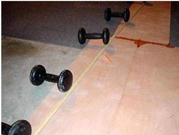
A batten being used to loft the deck.
